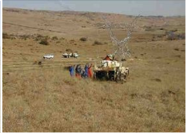
Stringing pilot cable with pilot tractor
