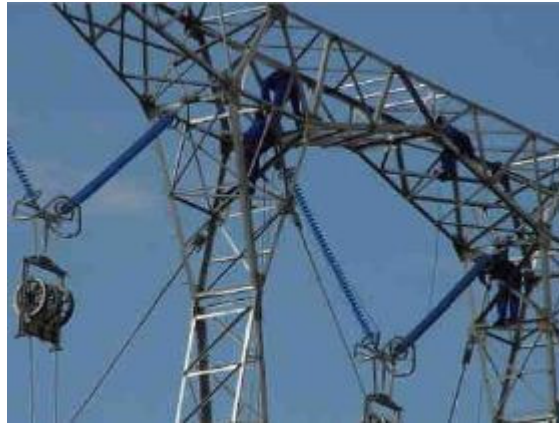
Using pulleys to hoist cable
