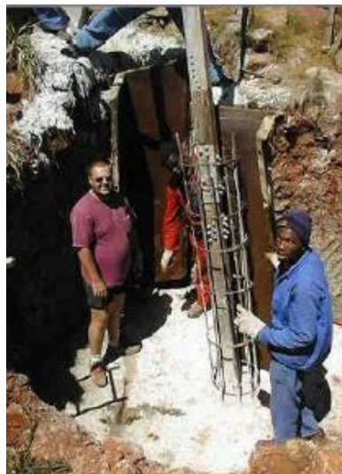
Foundation steelwork
