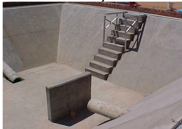
Example of an oil holding dam
